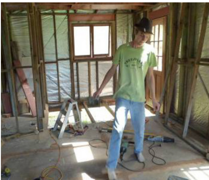
Taylor Logsdon helping with construction.
